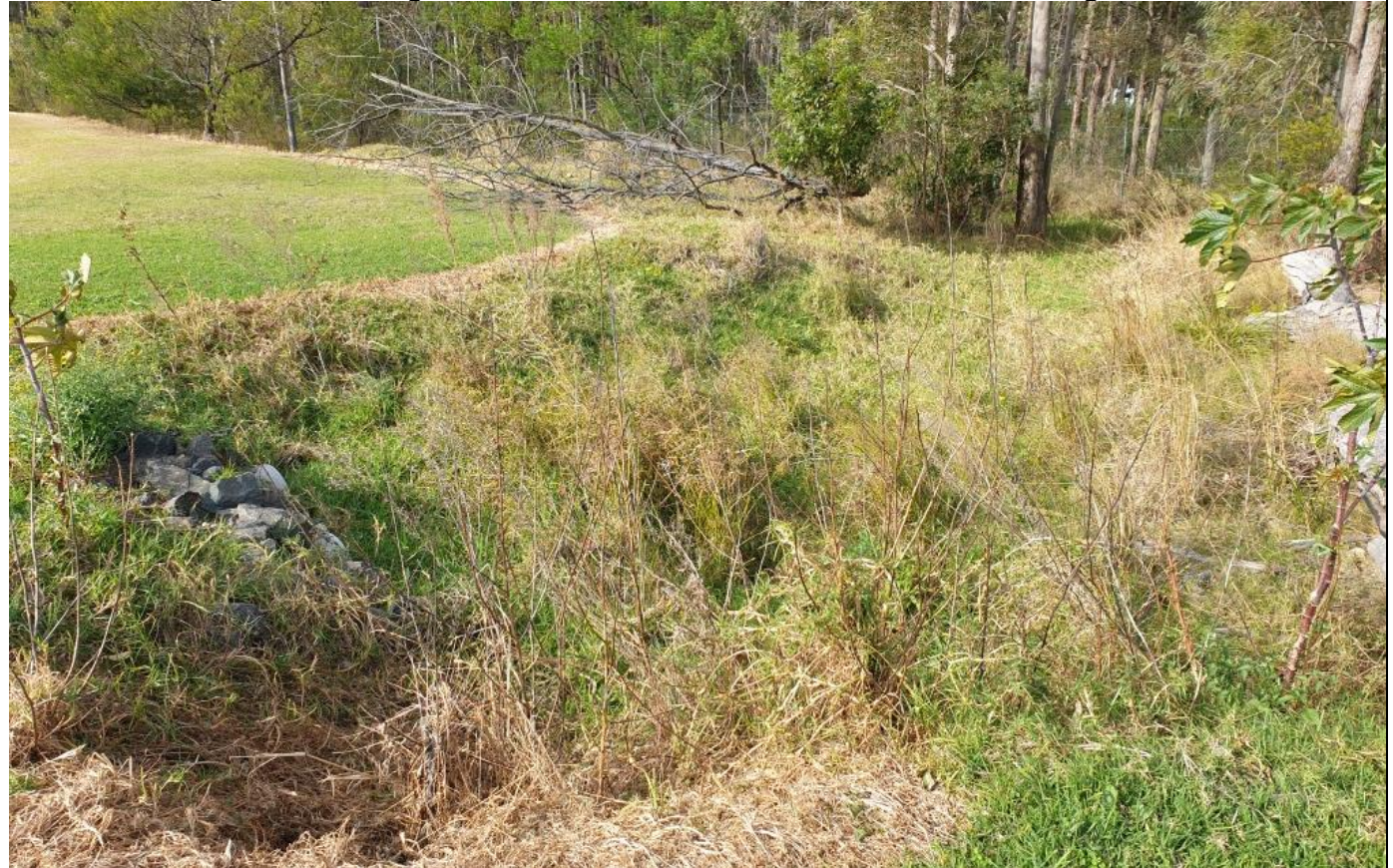
Photo 2. Existing central drainage outlet between fields 1 and 2, to Flinders Rd via vegetated swale
