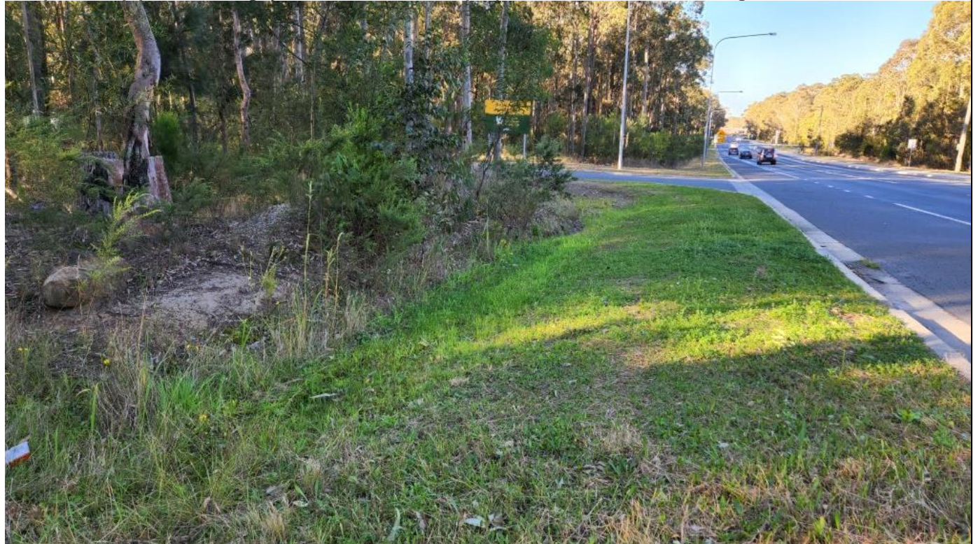
Photo 6. Flinders Rd verge where stormwater from the Rugby Park central drain currently discharges to and pools. A pipe under Rugby Park access road is proposed to connect to existing eastward table drain
