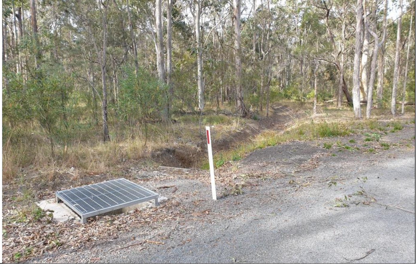
Photo 5. Existing pit and tail-out drain on access road, discharging onto neighbouring land – no increase in discharge would occur
